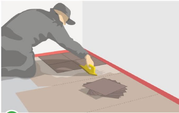
3 Final floor application (glued)
