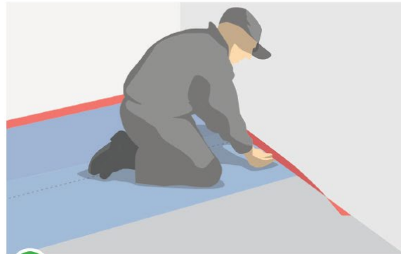
2 Perimeter barrier application
